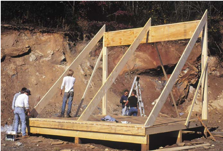
Above: Setting up 2 by 12 south wall rafters.
