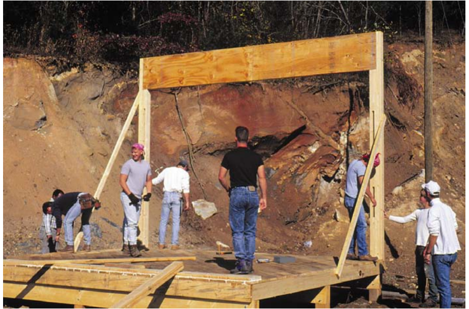
Above: Bracing the north wall.
