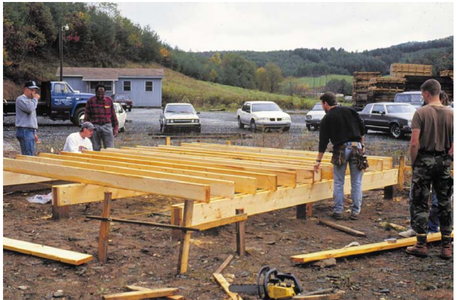
Above: Laying out foundation and floor.
