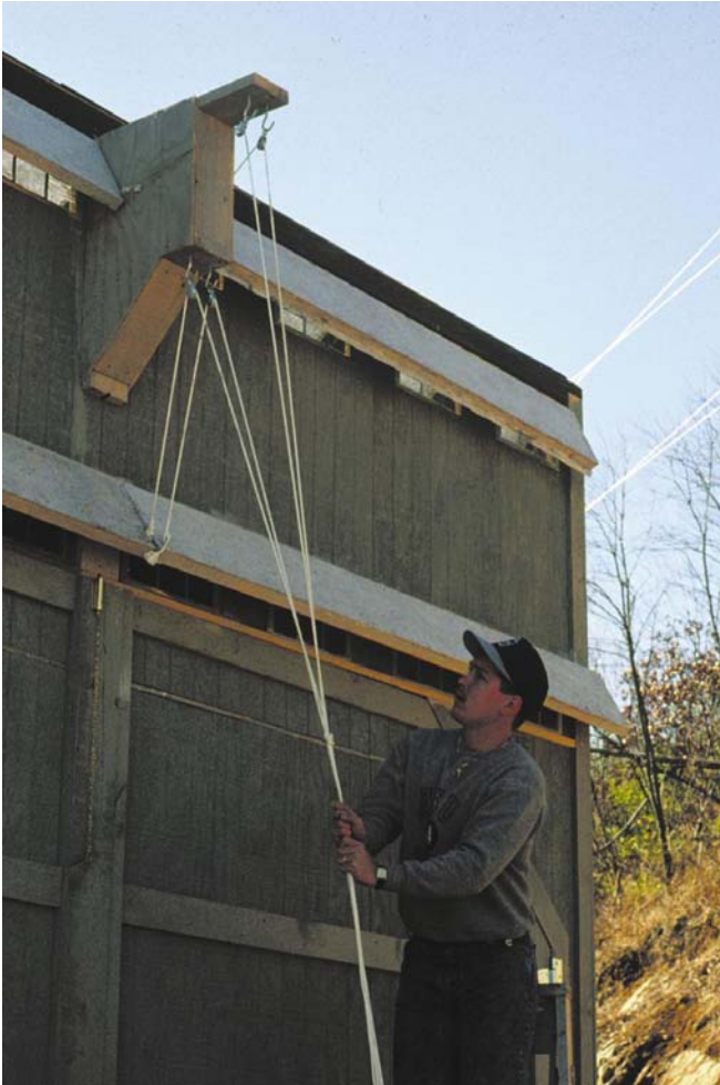
Above: Setting up vent control lines.
