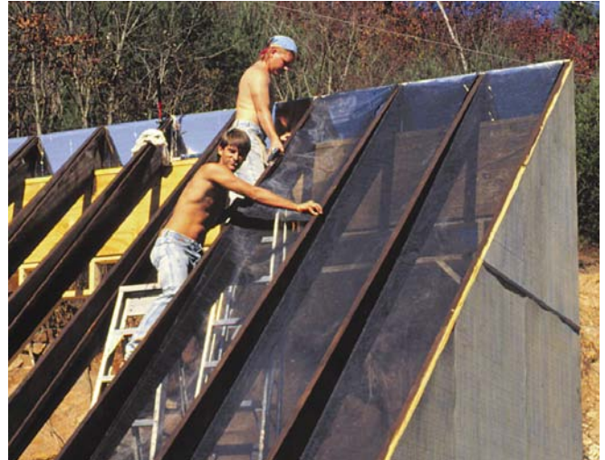
Above: Installing the dark aluminum screen used for solar absorption.
