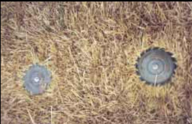
Old circular saw blades and threaded rod tie connecting interior walls to the straw.
