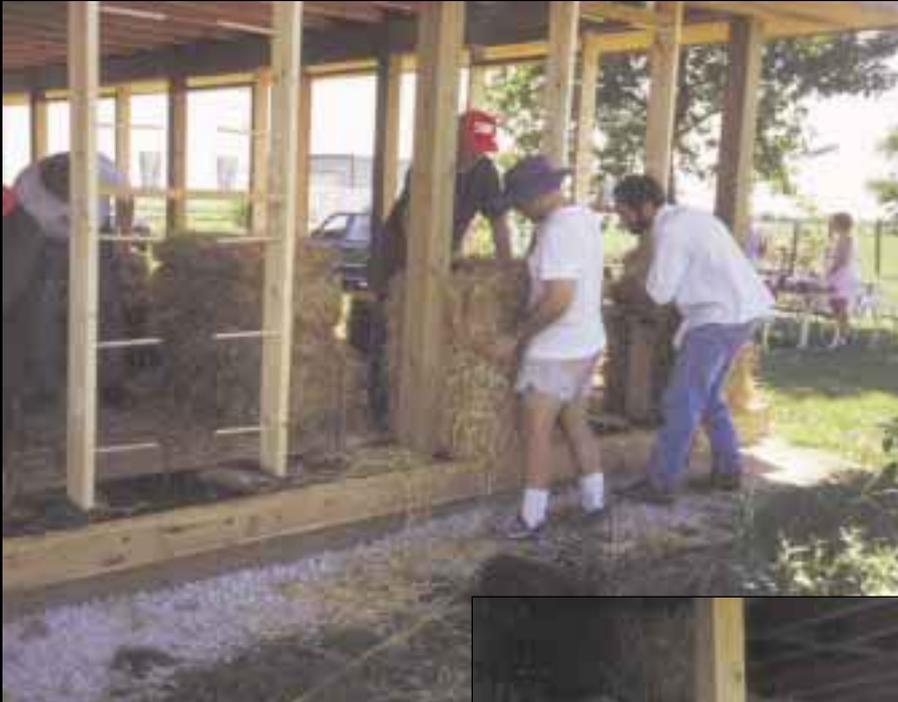
Stacking bales begins. Some bales were cut and retied to fit between posts and window frames.
