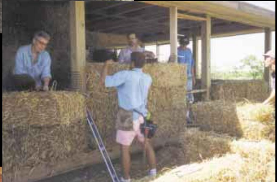
Interior walls are 2 by 4s, framed 24 inches (61 cm) on center. Both the slab floor area and the wood floor over the cellar are visible.
