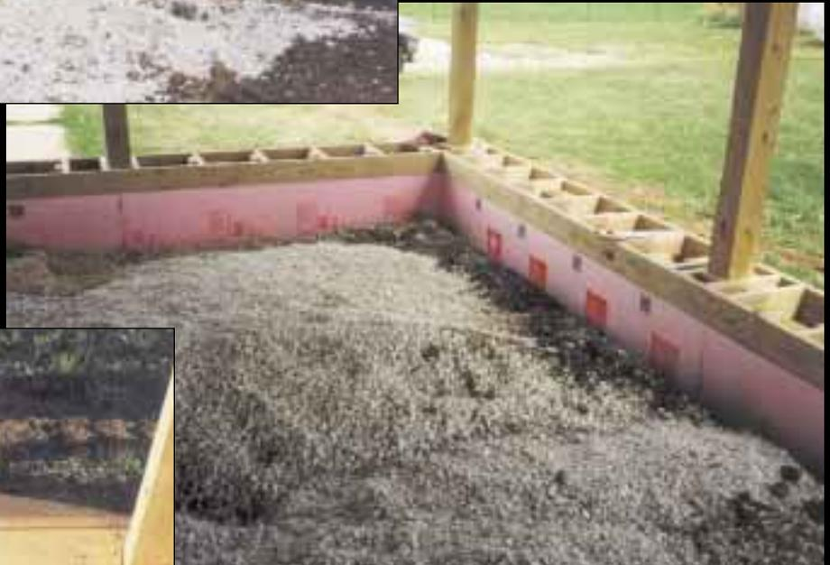
I built a frame to support the straw around the perimeter of the slab, to be consistent with the other foundation-to-wall detail.
