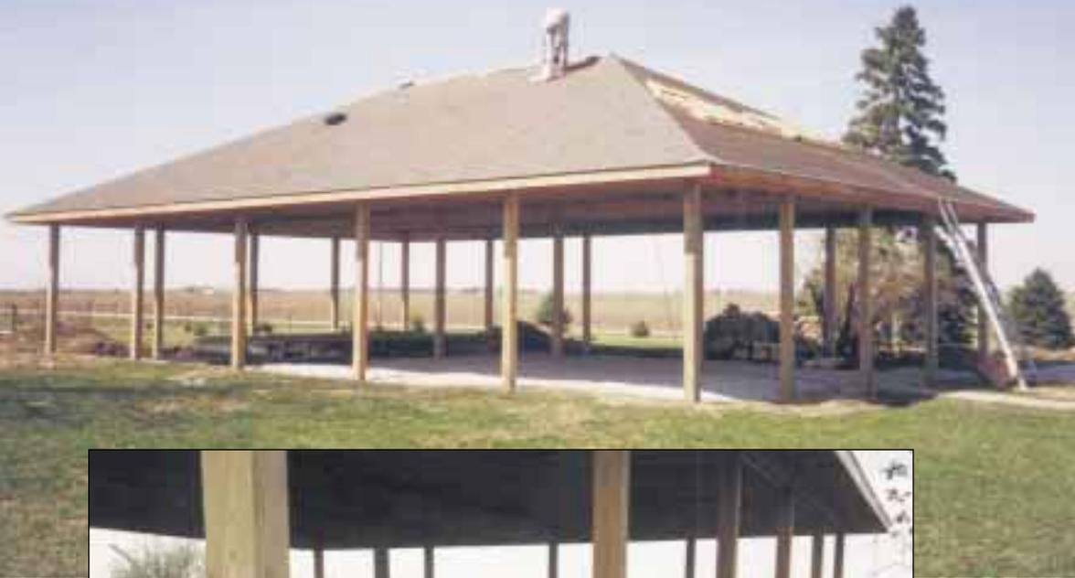
The framed hip roof has a 6/12 pitch with 2 foot (0.6 m) overhangs.
