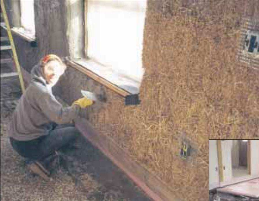
For wiring in the straw, we used BX cable and metal boxes screwed to wooden stakes. Main wire runs are in the attic.
