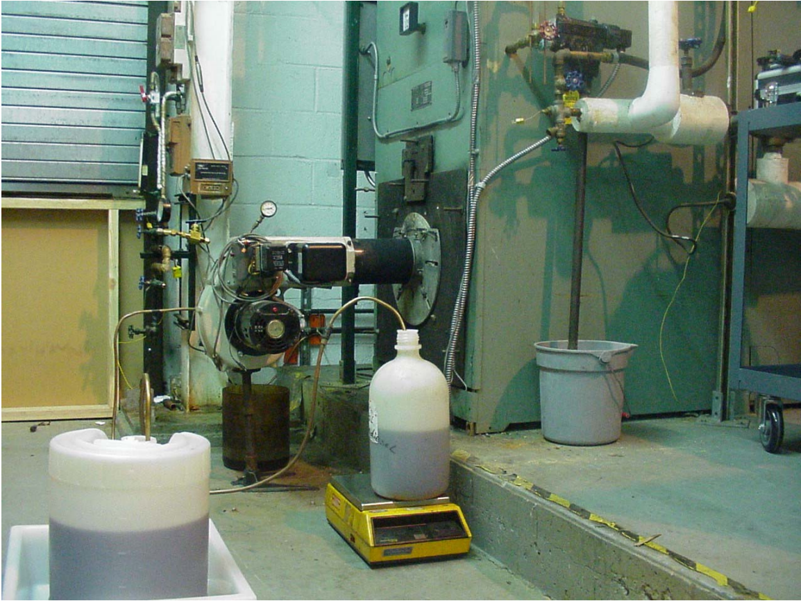
Figure 2. Commercial Boiler Set Up
