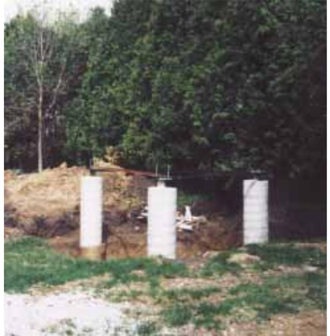
**Three concrete and rebar piers, poured around 8 foot angle iron legs, are embedded in the foundation.**
