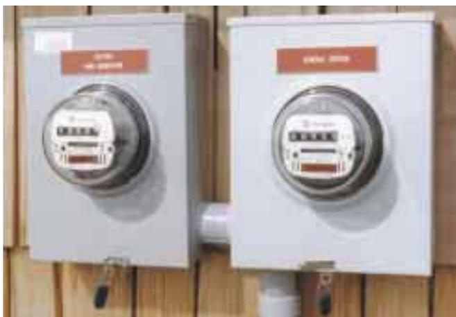
Above: Our detent meters. Service meter on right measures inflowing power. Wind Generator meter on left measures outflowing power.
