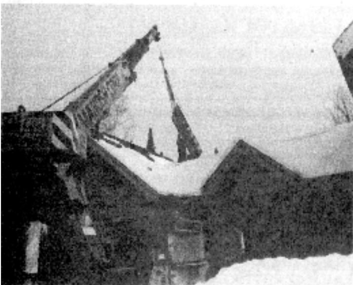
Using a crane to install the trackers with PV modules already attached and wired. Photo by Jay Kennedy, Village Photographer.
