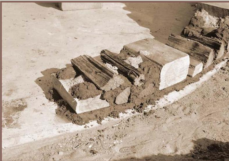
The timesaving building mantra is: Mortar. Insulation. Wood. Using your gloved hands, grab a glob of mud and plunk it down on the foundation, about an inch thick. (If your MIM stick is made from 1-inch-thick material, it can double as a mortar depth-checker!) Keep adding more mud, extending the 4-inch-wide (10 cm) mortar bed for 3 or 4 feet (91–122 cm). Now do the same thing for the other parallel mortar bed.
